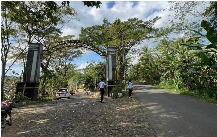
Figure 0-17 Access Road to TPA Sanggrahan
