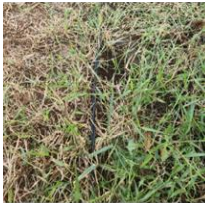
Electrical cable network near WWTP and active waste pile
